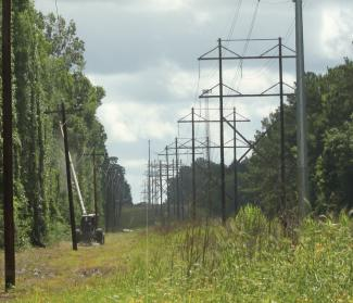
Right-of-way is the area around and below the power lines. Natchez Trace Electric clears this area of trees, limbs, and other vegetation to reduce the number of power outages and lower the risk of someone coming into contact with the power lines.
